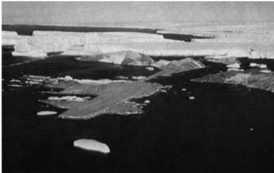
Figure 118. Runway at Dumont d'Urville during construction (1990). This view is from the seaward (northwest) end. At this stage of construction, Ile Cuvier and Ile du Lion had been leveled and the pass between them had been filled. The islands at the southeast end (Iles Buffon) were still awaiting leveling when this photo was taken. The ice in the background is the tongue of the Glacier de l'Astrolabe. (Photo courtesy of Michel Engler, Expéditions Polaires Françaises.)
